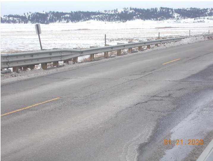
View of bridge H-13-N looking northeast.
