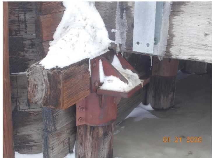
Paint sampled as H-13-N-LP01. The brown paint does not contain lead.
